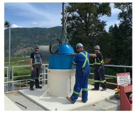
Fig 3. Fish Friendly pump installation at Pitt Polder P.S.
