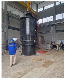
Fig 2. Pump onsite for instal
